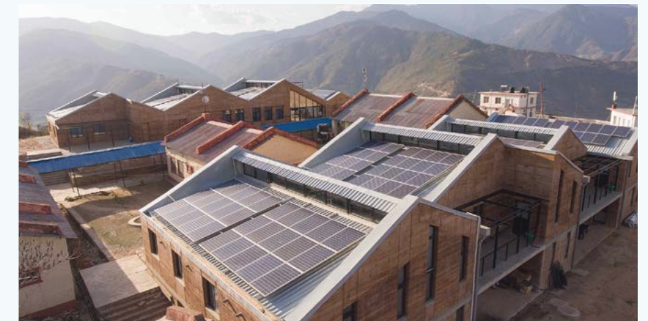
An aerial view of solar panels installed by SunFarmer Nepal at Bayalpata
